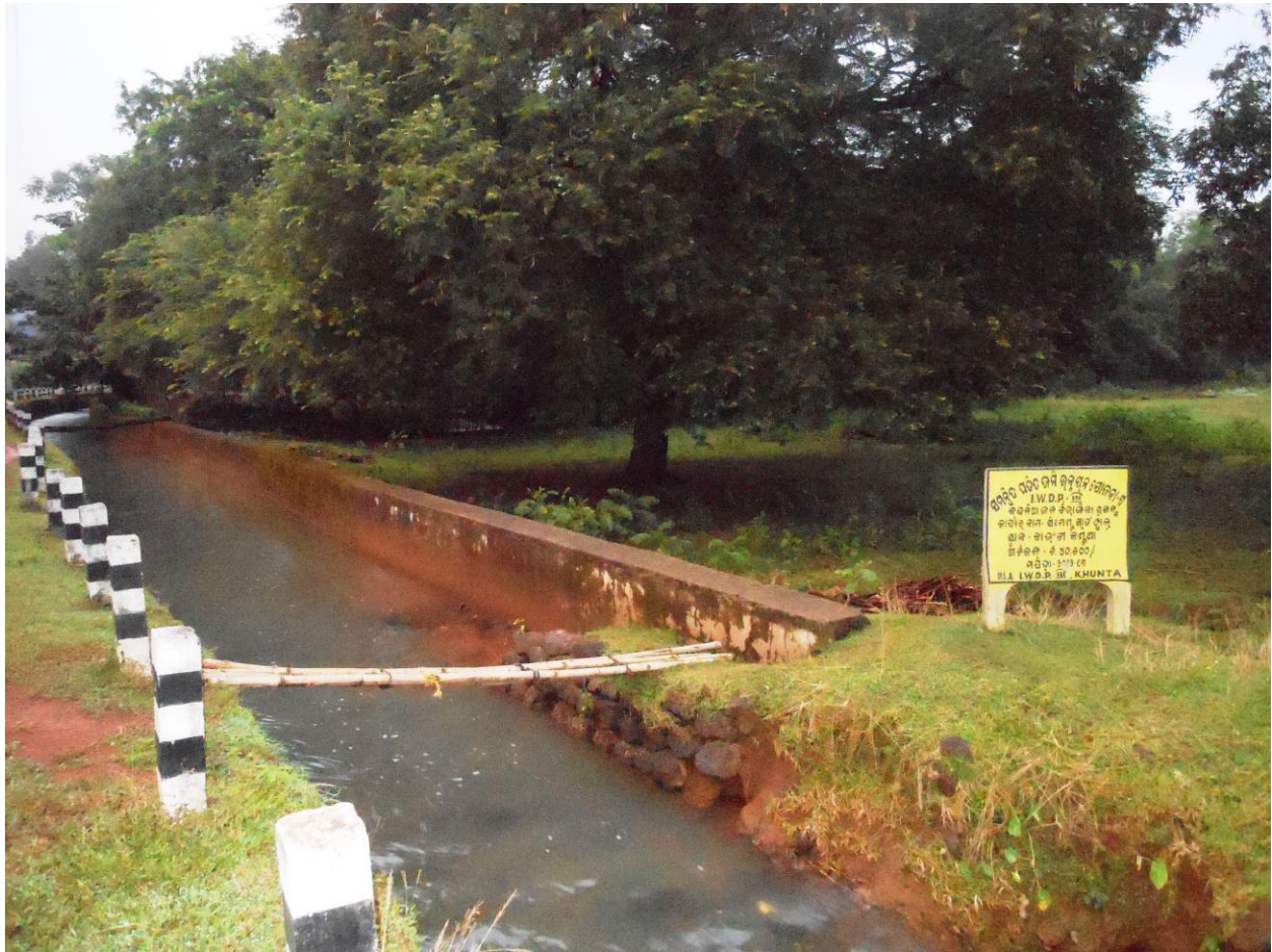
Integrated Wasteland Development Project(IWDP) has been implemented in India in several phases. This cement guard wall has been constructed in a village of Mayurbhanj district under this project.
